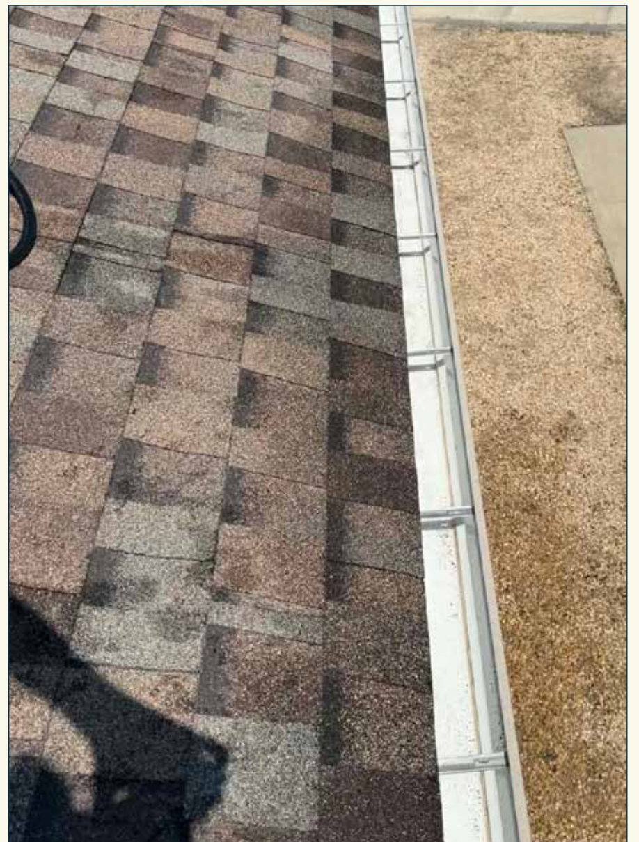
Before and after: Cleaning out eavestroughs is one of the fall maintenance jobs that can help prepare a home for the winter months. Removing leaves and debris allows water to drain properly and helps prevent potential problems when snow and ice arrive.
